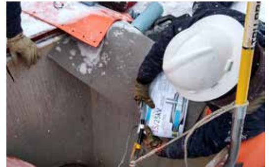
Figure 1: Checking measurements against MIC craftwork template during vault installation.
