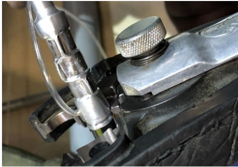
Fig. 4. Injection connectors are installed at each cable end to create a fluid access point for injecting silicone gel into the cable's conductor.
