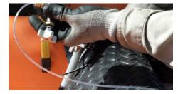
Our engineers have developed a revolutionary new process of injecting silicone fluid down the interstitial region in strand-blocked conductors. This patent pending-process allows for the dielectric enhancement of all stranded conductor cables in the ground. Failing strand-blocked cables no longer have to be replaced. The Southwire® process allows strand-blocked cables to have their life extended with silicone rejuvenation.
