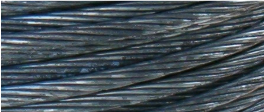
Figure 4. Oxidation on a conductor.
