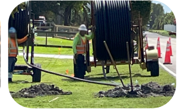
The CIC reel on the left was the first reel used for the pull. The reel on the right was staged for the second pull for the next segment.
