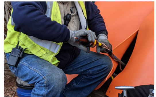
Figure 1: Assembling the MIC body onto the cable.
