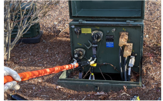
Figure 3: Completing MIC Injection.
