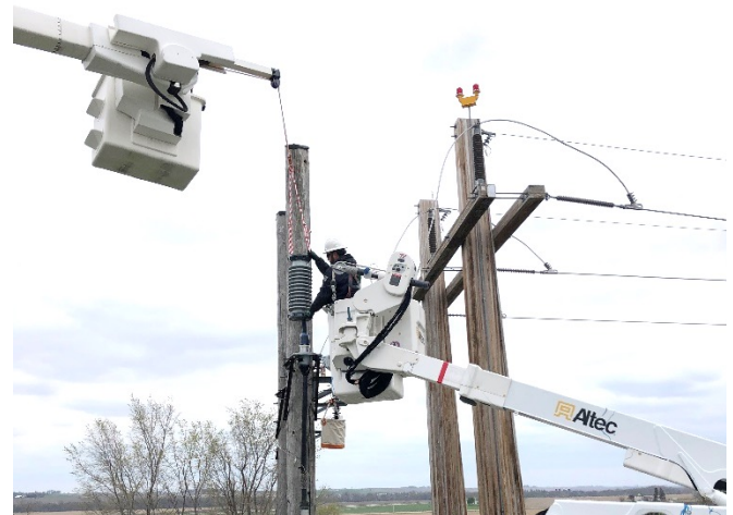
Figure 4: Lifting the porcelain body into position using jib crane.
